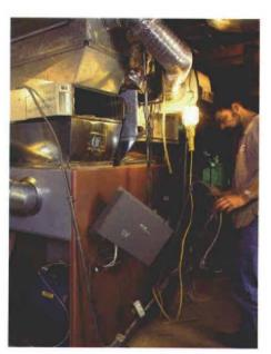
Forced-air systems offer varied climate control. Hot air delivered from this oil-fired furnace isn't the only use for a forced-air system. It's also used for air conditioning, ventilation, humidification and air filtration.
