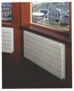
Low-profile radiators need little space. Installed along the exterior walls, baseboard radiators use radiation and convection to heat a room. Air flows upward through the hotwater heated radiator, warms and rises to heat the room.
