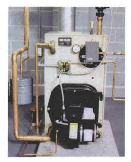
**Oil-fired furnaces have become more efficient.** This oil boiler has an efficiency rating of 84% or better. Most oil furnaces and boilers on the market today have annual fuel-use efficiencies in the range of 78% to 82%.
